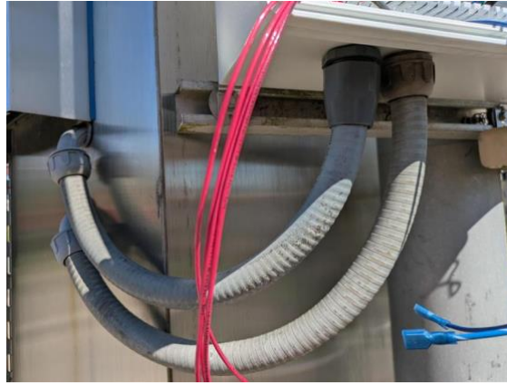
Example of how to run conduit from the bottom of the STREAMETRIC Enclosure to the Main Control Panel
